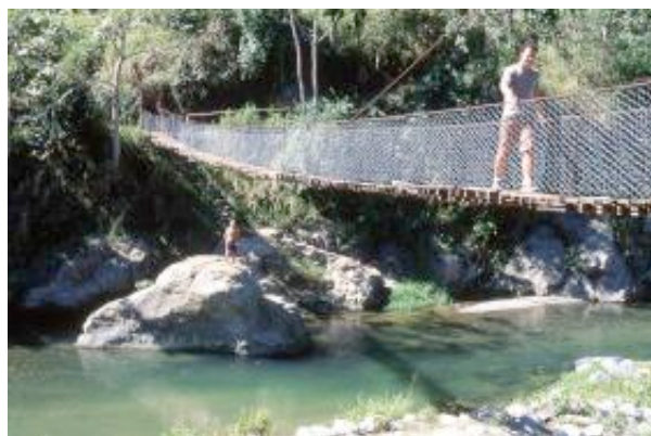
Crossing a bridge over a Dominican stream
